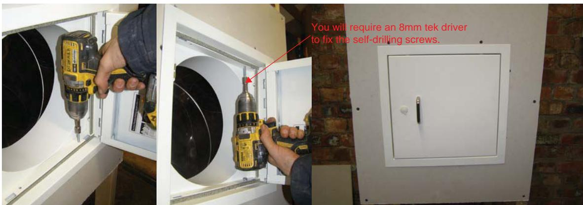
6. When you are ready to fix the chute door, offer it up and check alignment. Ensure the door frame is sitting flush against the finished wall while the door is open.
