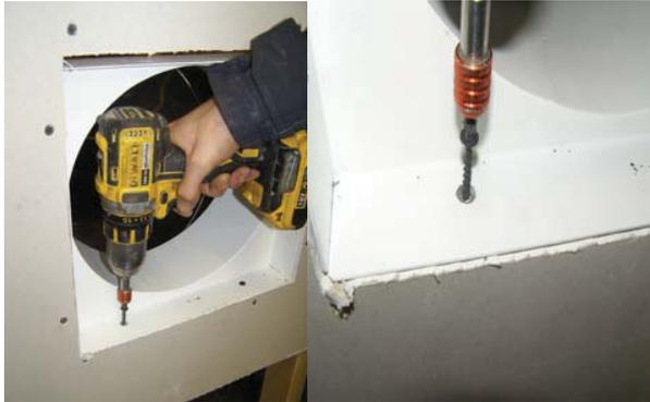
5. Fix the frame into the stud-work opening through the fixing holes using the screws supplied.
